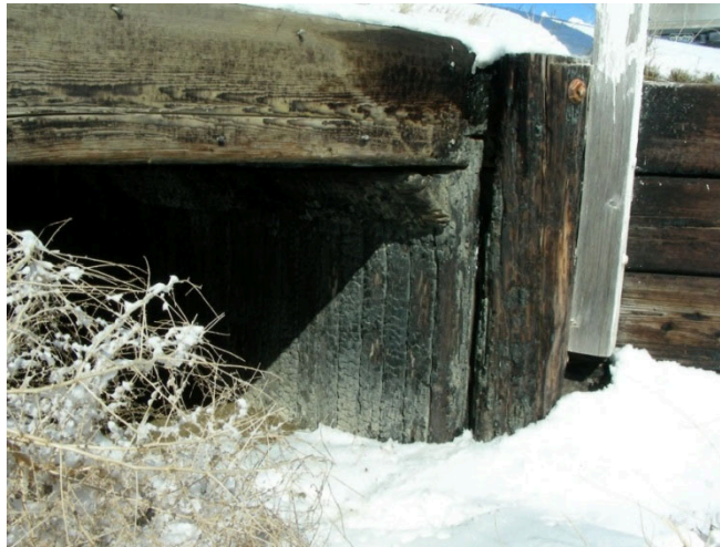
Figure 4.13.2-6—Fire Charring on Timber Culvert Members
