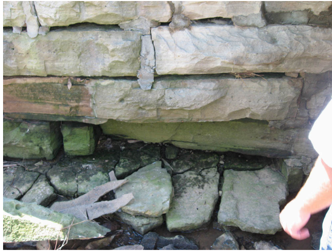
Figure 4.12.2-1—Missing Units in Masonry Barrel Wall with Cracked and Missing Mortar
