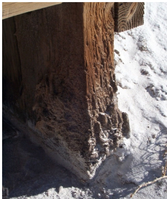
Figure 4.13.2-3—Decay on Timber Culvert Member near Ground Level
