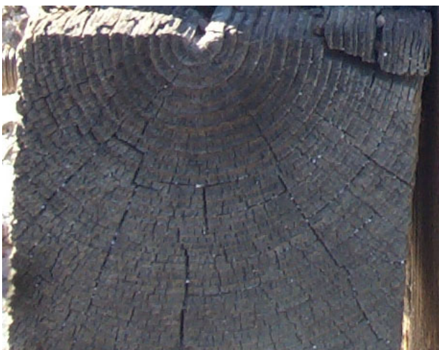
Figure 4.13.2-7—Checks in Timber Culvert Member
