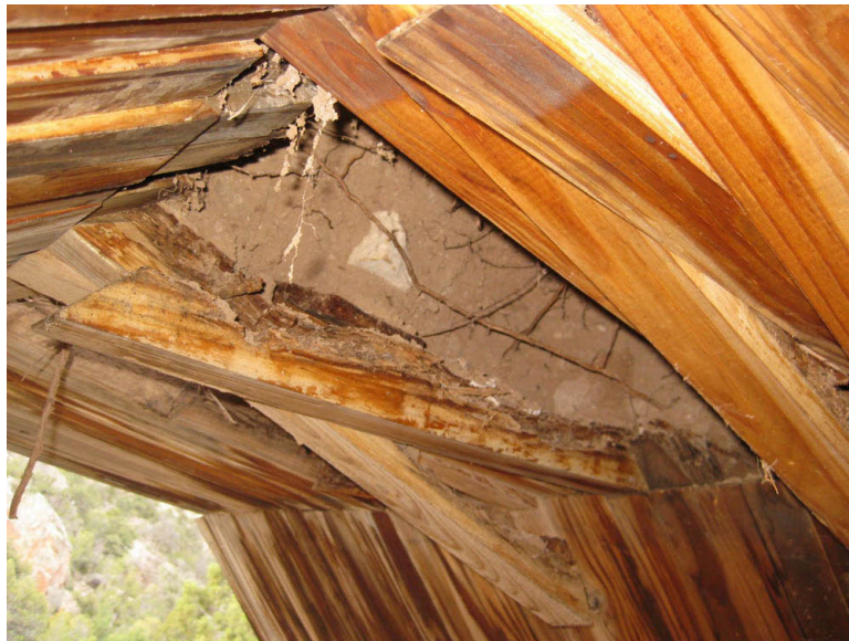
Figure 4.13.2-2—Connection Failure Causing Partial Collapse of Member and Missing Members Allowing Loss of Backfill
