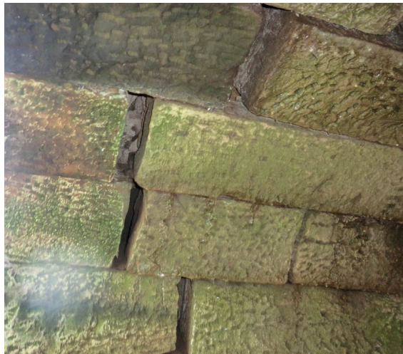
Figure 4.12.2-3—Missing Mortar between Masonry Units
