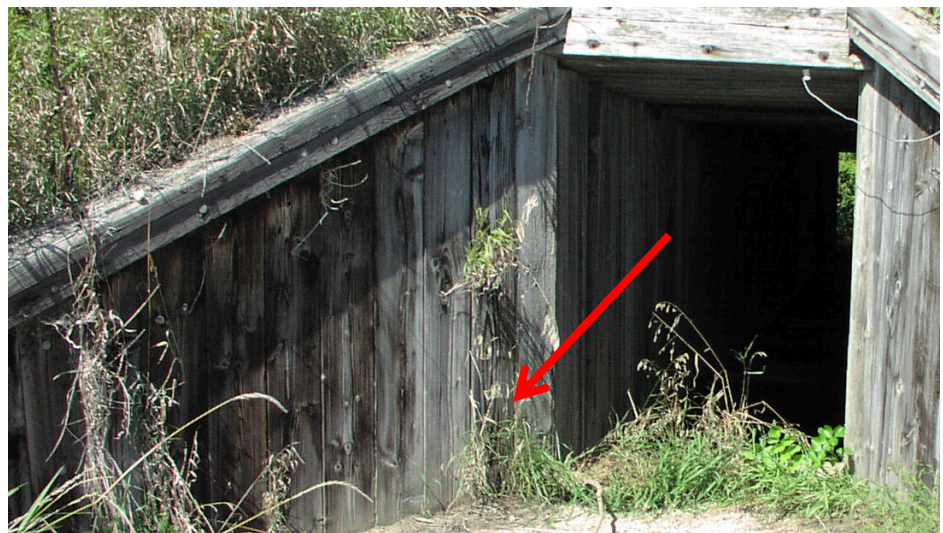
Figure 4.13.2-5—Staining and Sunken Faces on Timber Culvert Members
