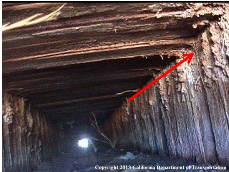
Figure 4.13.2-4—Fruiting Bodies on Timber Culvert Members
