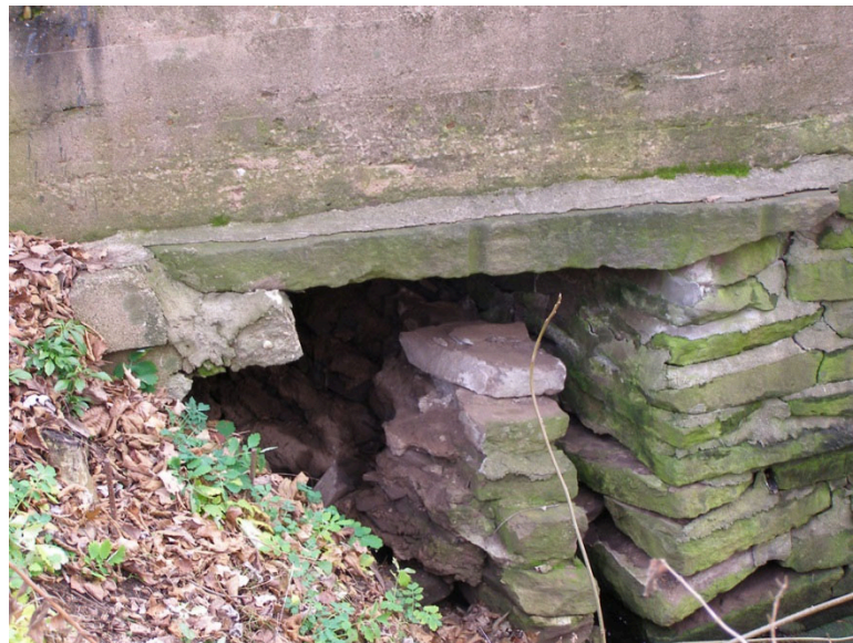
Figure 4.12.2-2—Structure Condition is Severe and Unstable Due to Movement of Foundation Wall
