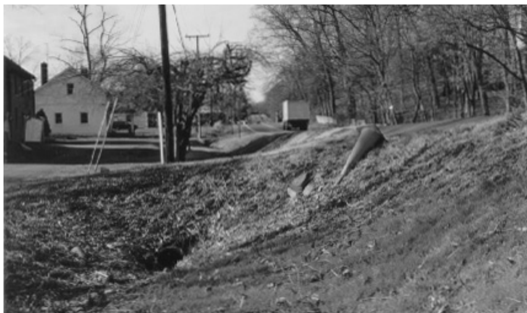
Figure 4-2. Undesirable steep slopes, both parallel and perpendicular to the highway.
