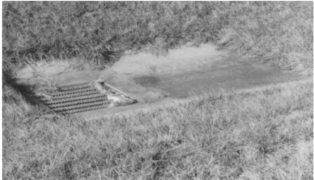
Figure 4-3. Traversable drainage inlet.
