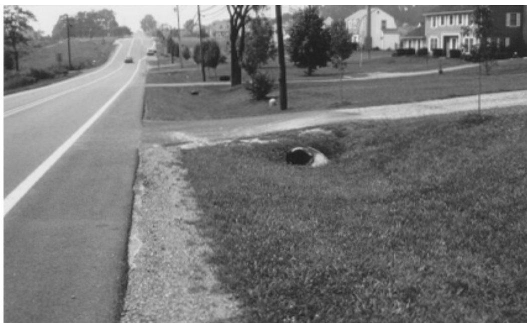
Figure 4-6. An errant vehicle can be guided by a ditch into a culvert opening even though outside the clear zone.
