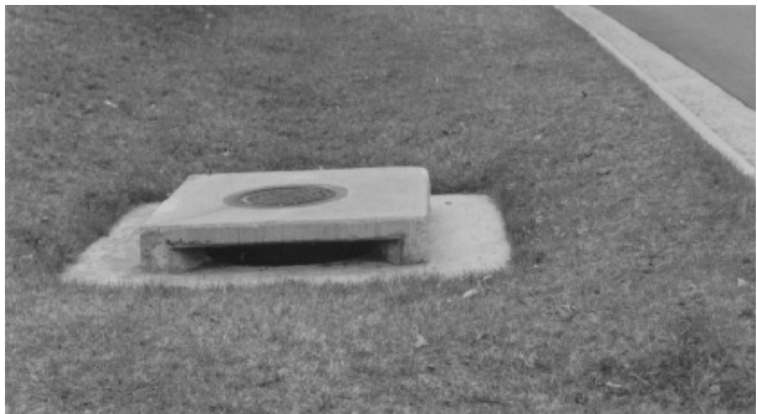
Figure 4-4. Existing inlet projecting more than 100 mm above the ground.
