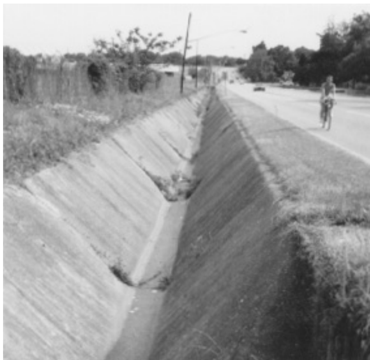
Figure 4-5. Nontraversable ditch.
