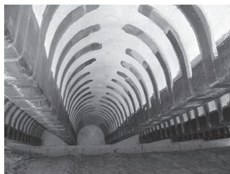
(b) Wet-Layup System (span B)
