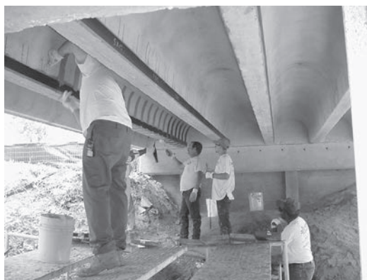
Figure 5—Strengthening of Span with Pultruded Plates
