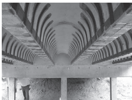
(a) Pultruded Plate System (span A)
