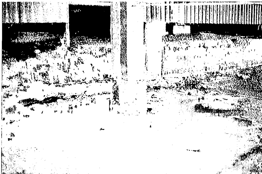
Fig. 8a—Rapid and severe corrosion damage of conventional construction materials in potash fertilizer plant areas exposed to both acid and salt solution
