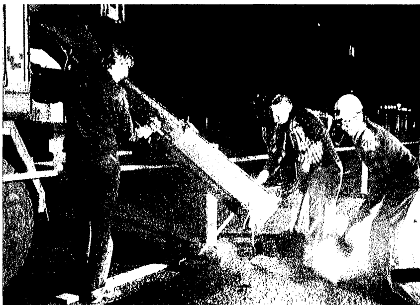
Fig. 15—SC can be used to complete road repairs overnight to reduce public inconvenience
