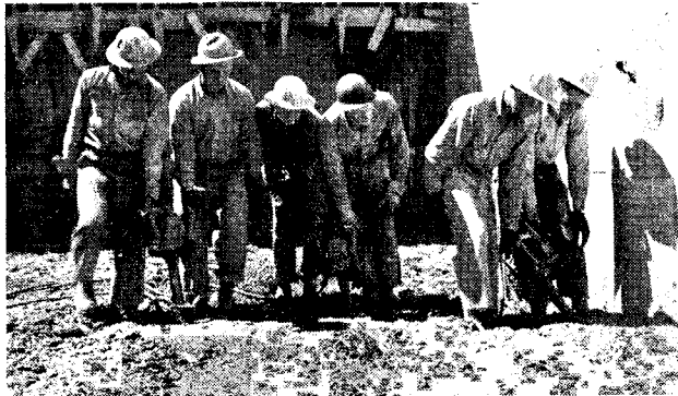
Fig. 5—The same concrete shown in Figure 4 as the vibration nears completion
