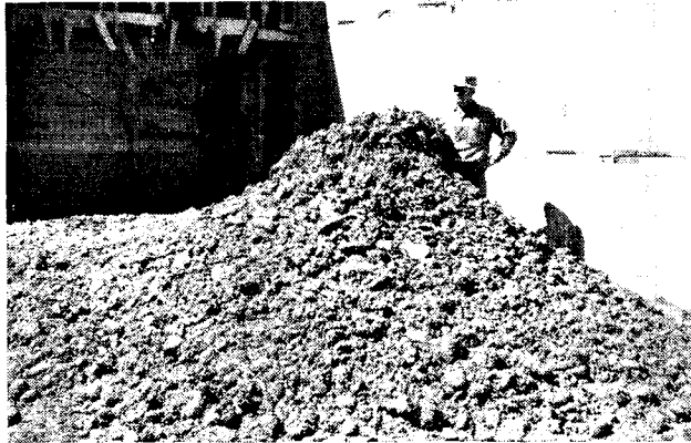
Fig. 4 — Eight cubic yards of concrete immediately after dumping from cableway bucket and before vibration
