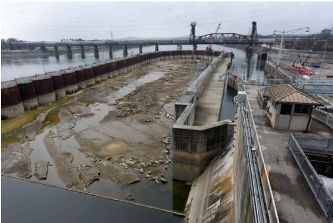
Figure 6 —Rust Stains and Efflorescence Visible (Right Side) During the Chickamauga Lock Replacement Project in Tennessee (Source: U.S. Army Corps of Engineers)
