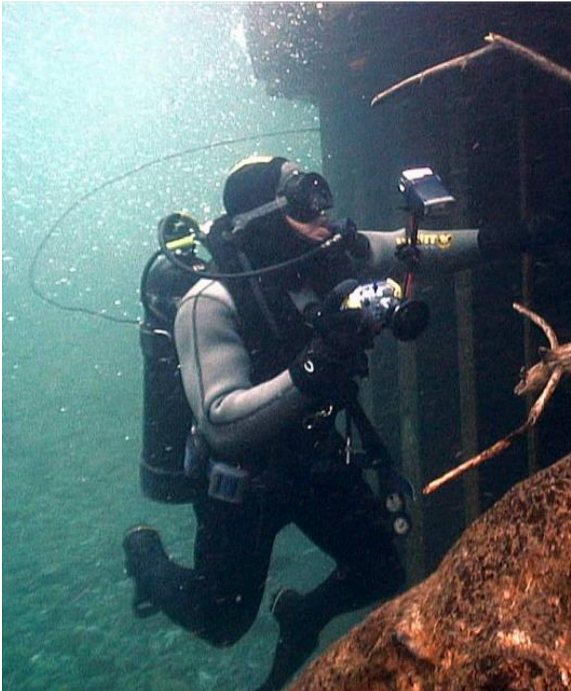
Figure 7 —A Diver Taking a Photograph of a Bridge Substructure with a Digital Camera in Waterproof Housing (Source: Federal Highway Administration [19])
