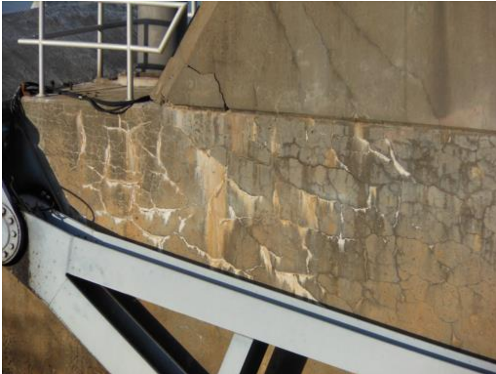
Figure 5 — ASR Damage in a Dam Pier at David Terry Lock and Dam in Pine Bluff, Arkansas ( Source: U.S. Army Corps of Engineers )
