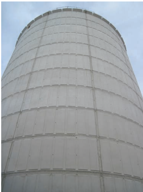
Fig. 14.13: Visual pattern formed in cast-in-place water tank structure (Photo courtesy Landmark Structures)
