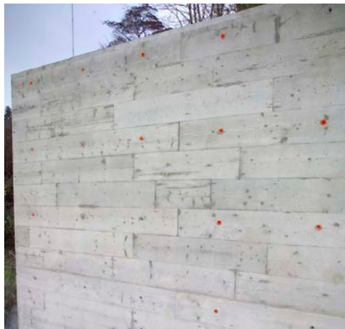
Fig. 14.19: Wood board sheathing joint and grain pattern (Photo courtesy Doka USA)
