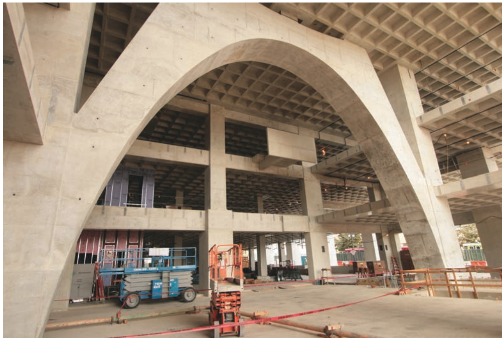
Fig. 14.28: Concrete arch and coffered two-way joist ceiling become major statements contributing to architecture (Photo courtesy Morley Builders)
