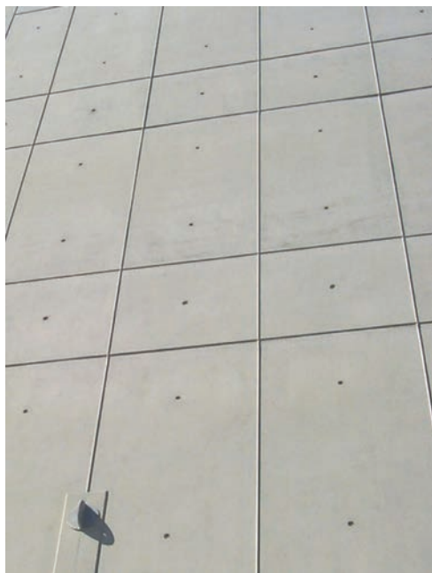
Fig. 14.21: Tie holes located to become part of the visual design (Photo courtesy Morley Builders)
