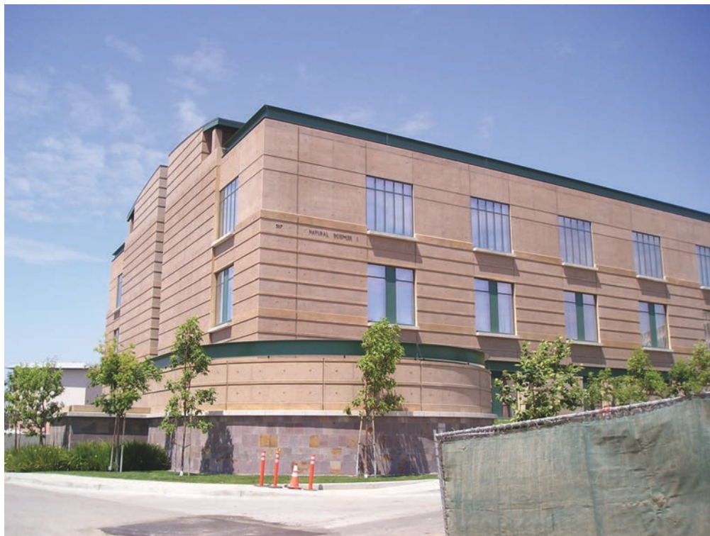
Fig. 14.11: Rustication joints create visual patterns (Photo courtesy Olympic Panel Products LLC)
