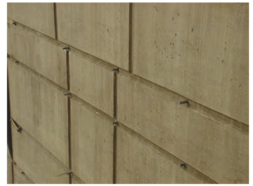
Fig. 14.22: Fiberglass ties colored to match concrete and aligned in rustication joints to further minimize visibility after final trimming is completed (Photo courtesy RJD Industries)
