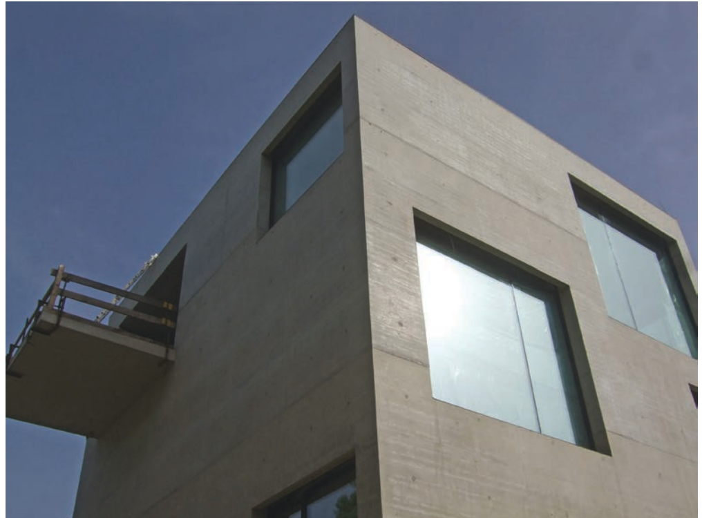
Fig. 14.23: Alignment and tightness of joints at corners and windows is critical in architectural concrete (Photo courtesy MEVA Formwork Systems)
