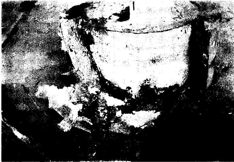
Fig. 5—Concrete pile cap showing severe sulfate attack causing overlay cracking
