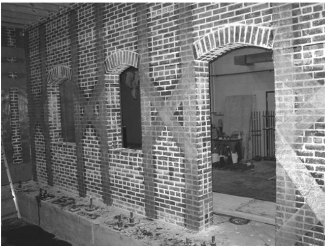
Fig. 10.2—Wet lay-up unidirectional glass fabrics with epoxy matrix (Moon 2004).
