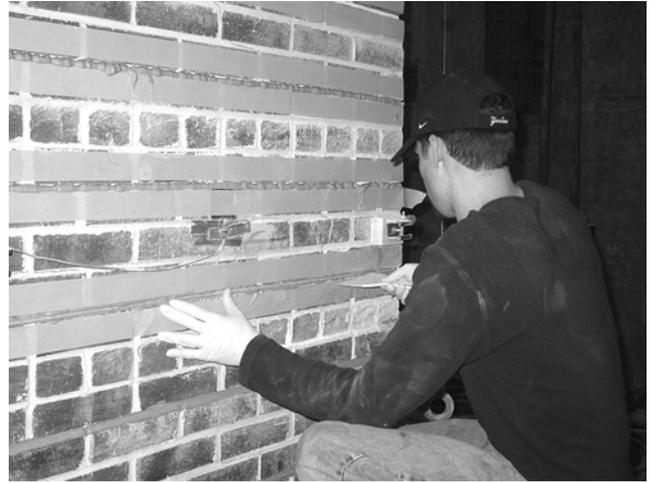
Fig. 10.3—Epoxy adhesive-applied NSM GFRP rods (Moon 2004).
