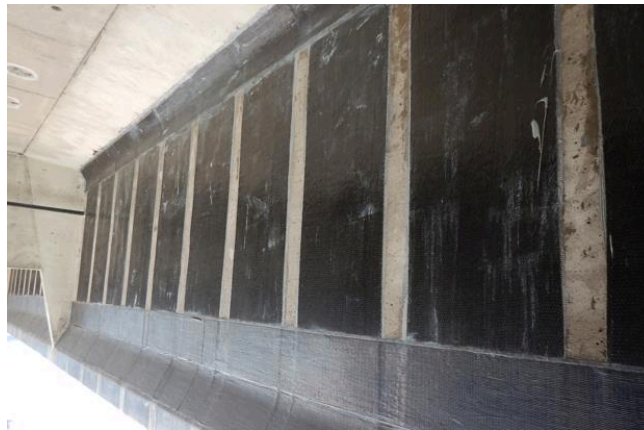
Figure 1 — Application of CFRP vertical shear strips and horizontal anchor strips on I-girders of the Champlain Bridge in Montreal (Courtesy of the Jacques Cartier and Champlain Bridges Inc.)
