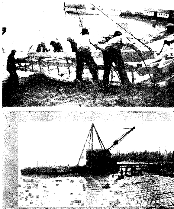
FIG. 11—PAVING UPPER BANK SHOWING MAT-LIFTING FRAME AND GRAPPLE HOOKS
