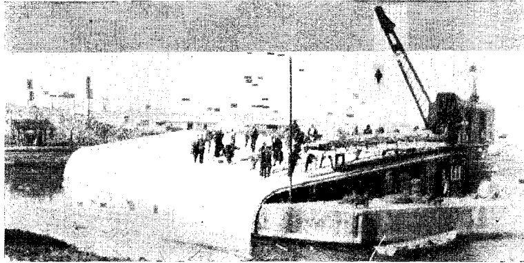
FIG. 9—PAVING UPPER BANK WITH FLOATING LOCOMOTIVE CRANE FIG. 10—ASSEMBLING MAT SECTIONS, SINKING BARGE (25 SQUARE LAUNCH)
