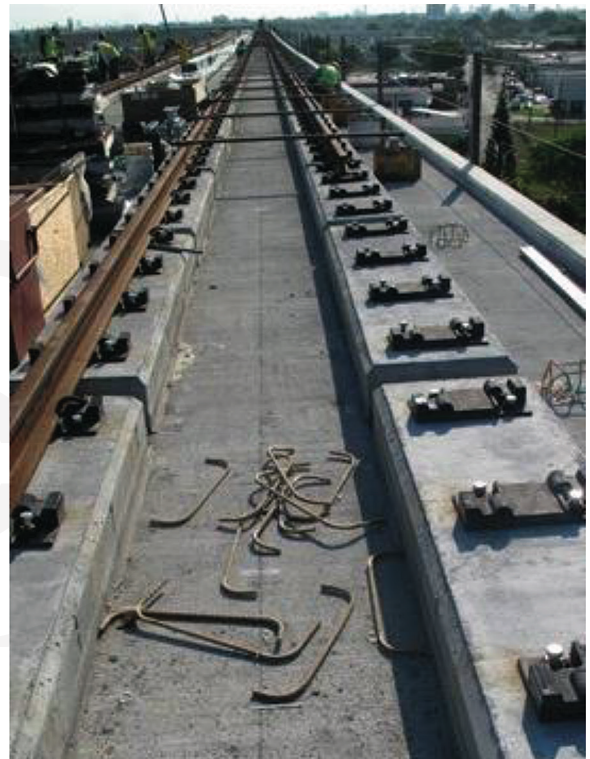
Fig. 3.2e—GFRP bars used in rail plinths.
