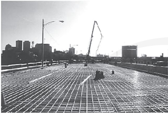
Fig. 3.2b—GFRP bars used in the redecking of Dayton, OH, Salem Avenue Bridge in 1999.
