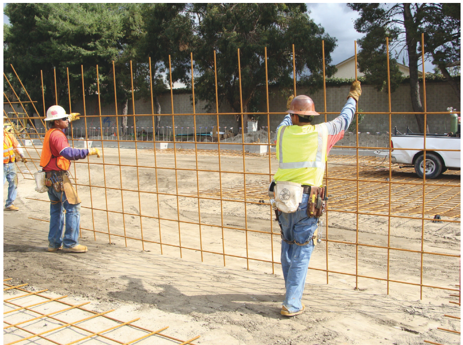
Fig. 8.21—Sheets of WWR with larger wire sizes spaced a minimum of 12 in. (300 mm) on center provide space for construction foot traffic. They also make it much easier to maintain the required depth of the reinforcement as compared to rolls of WWR with closely spaced wires. (Photo courtesy of Wire Reinforcement Institute.)
