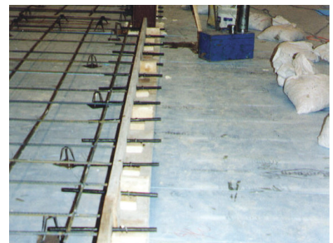
Fig. 8.23a—Dowels and welded wire reinforcement are supported in place. A contraction joint will be sawed above the dowels in the background of the photo that are located perpendicular to the construction joint. The welded wire reinforcement is stopped short of the joint.
