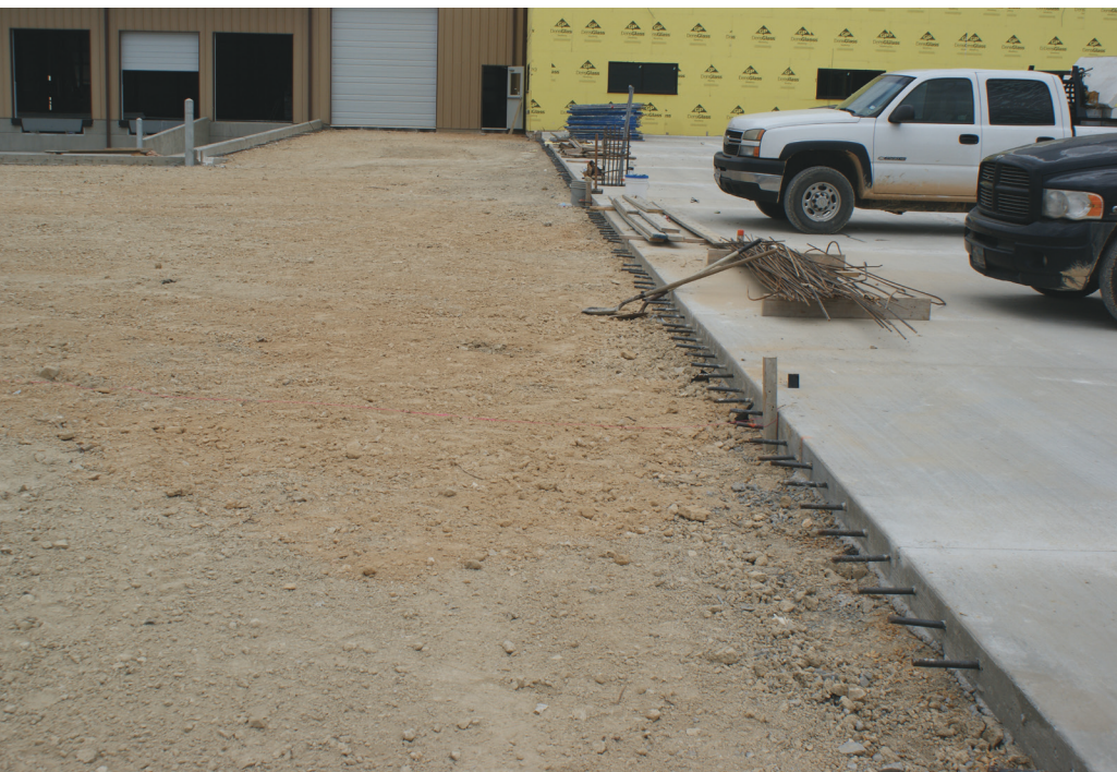
Fig. 8.23b—Dowels sticking out of concrete cast on one side of the joint.
