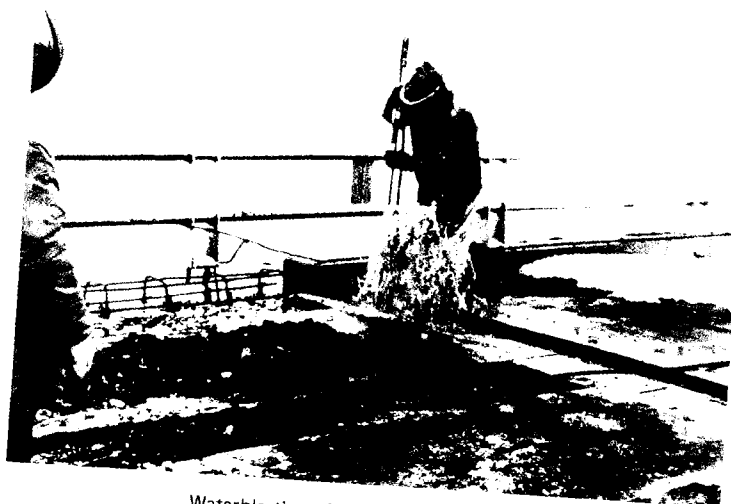
Waterblasting of Rubberized Tar Filler
