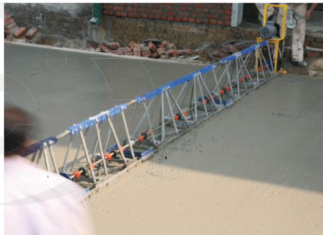
Fig. 3.2.4c—Vibratory truss screed.
