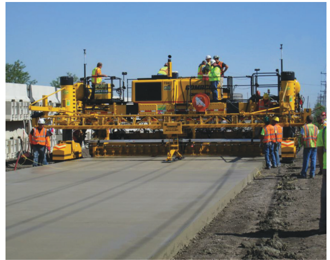
Fig. 3.2.4a—Slipform paver (courtesy of GOMACO Corp.).
