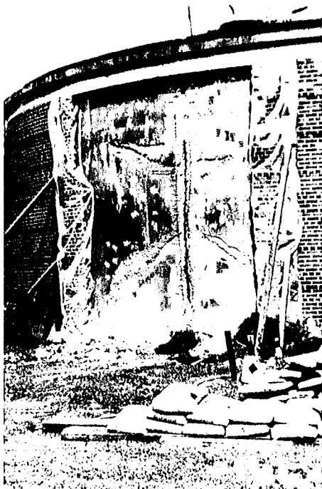
Fig. 10—Sewage tank failure
