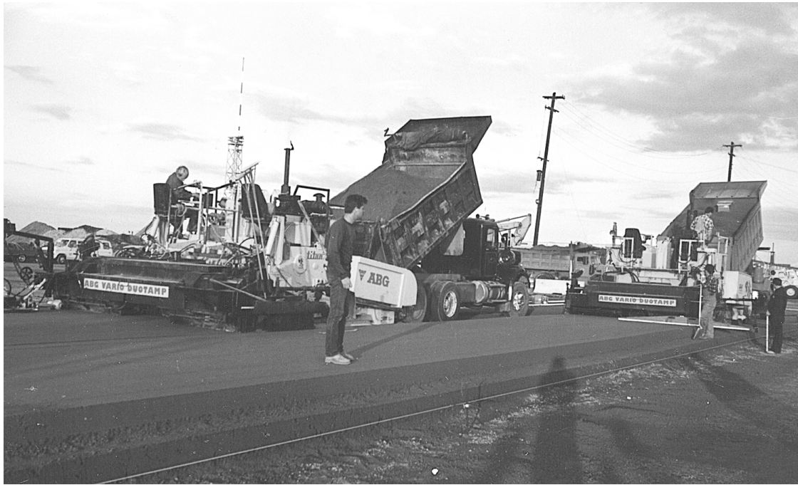
Fig. 2.1—RCC placement using modified asphalt pavers
