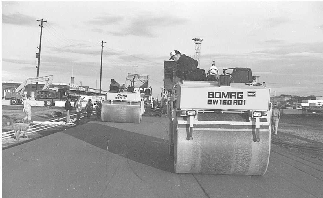
Fig. 2.2—Vibratory roller compaction
