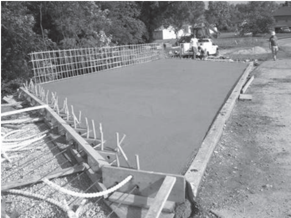
Figure 11—Poured FRP Bridge Deck
