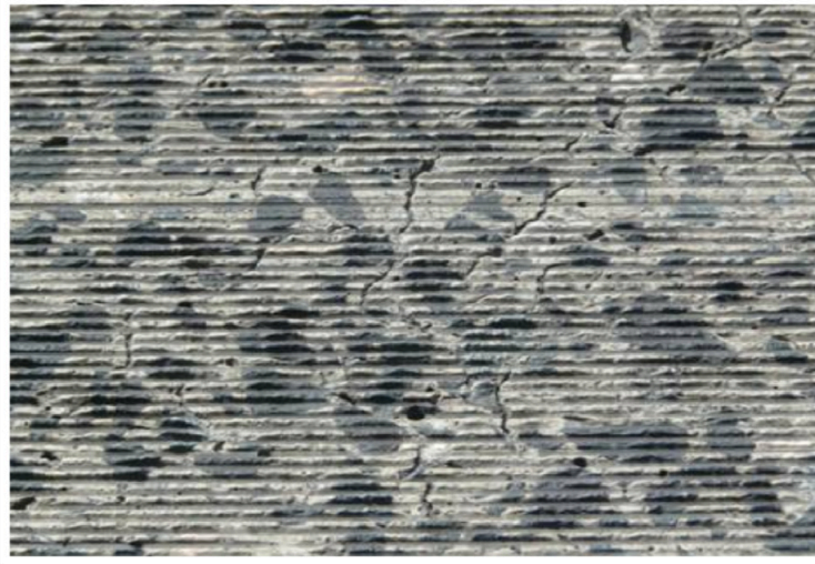
Figure 5 – Plastic shrinkage cracks
