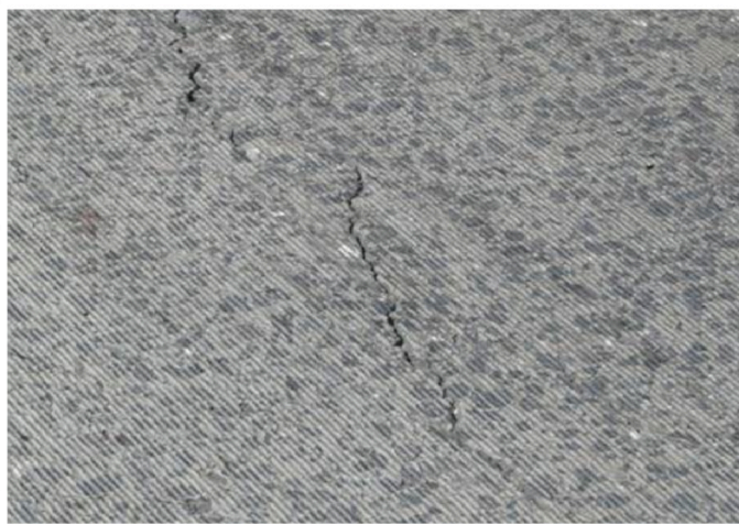
Figure 6 – Full depth cracks
