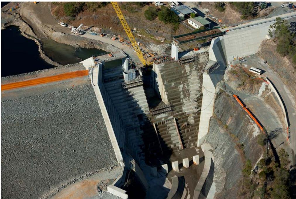
**Figure 2 – Aerial Photograph of Hinze Dam Spillway during Construction**
