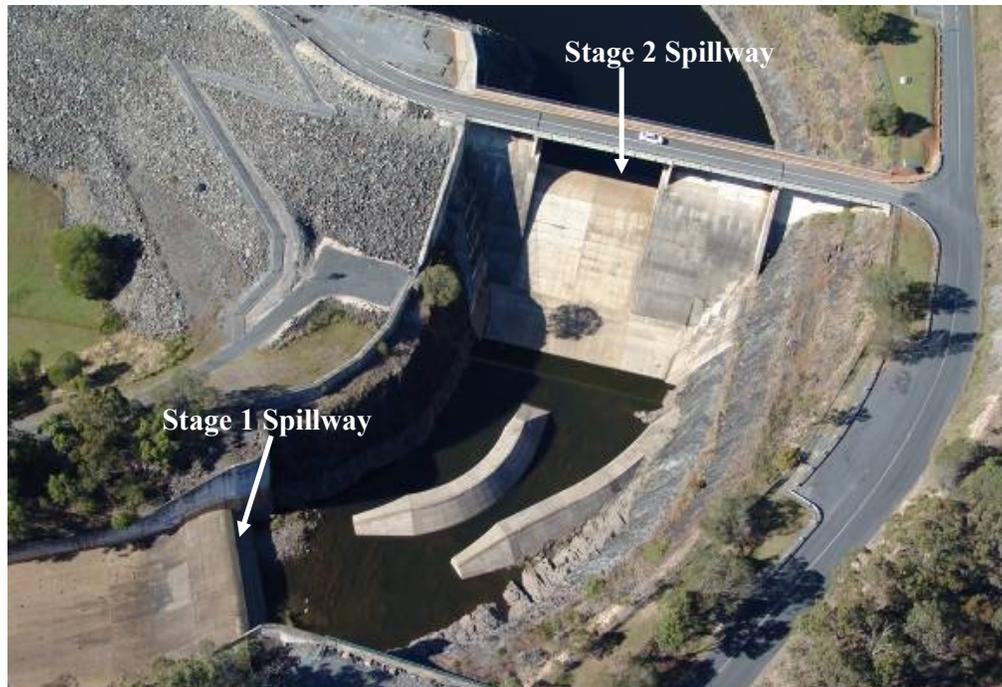
**Figure 1 – Aerial Photograph of Hinze Dam Spillway Prior to Construction**
