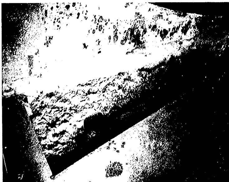
FIG. 8-2 PREPARED CAVITATED AREA ON WEST SIDE OF TUNNEL CENTER LINE. CORE HOLE AT LEFT CENTER
