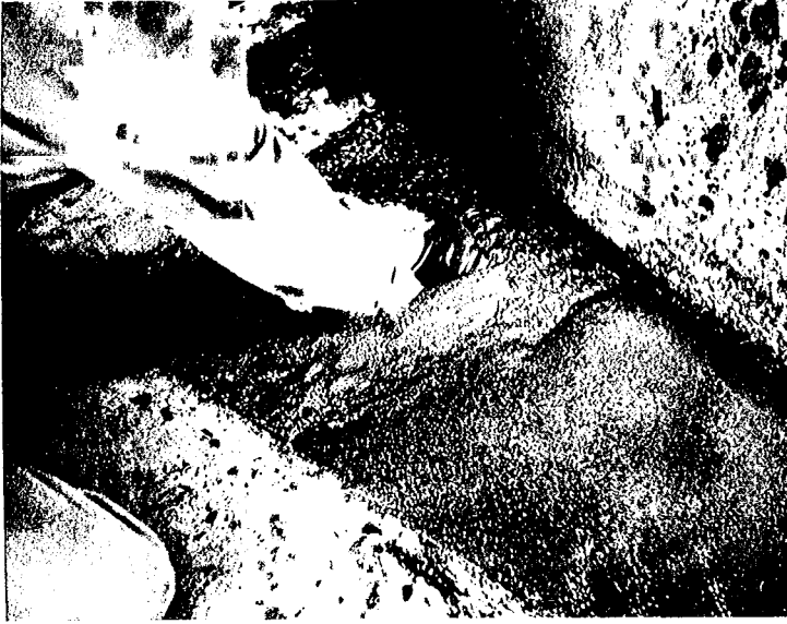
FIG. 8-3 PLACING EPOXY MORTAR OVER EPOXY CONCRETE IN WEST CAVITATED AREA
