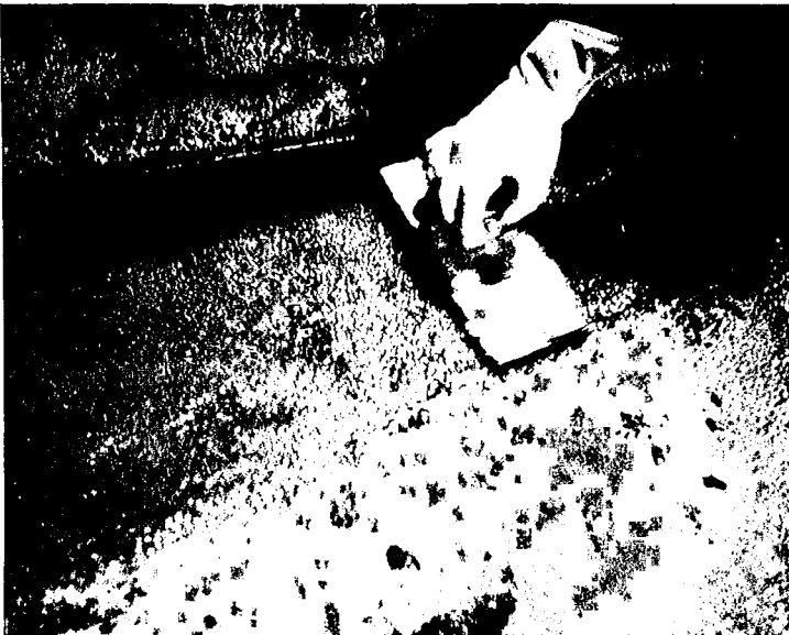
FIG. 8-4 FINISHING SURFACE OF EPOXY MORTAR IN WEST CAVITATED AREA
