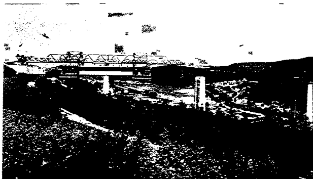
Fig. 28-37 - Half-Spans Nearing Completion at First Pier
