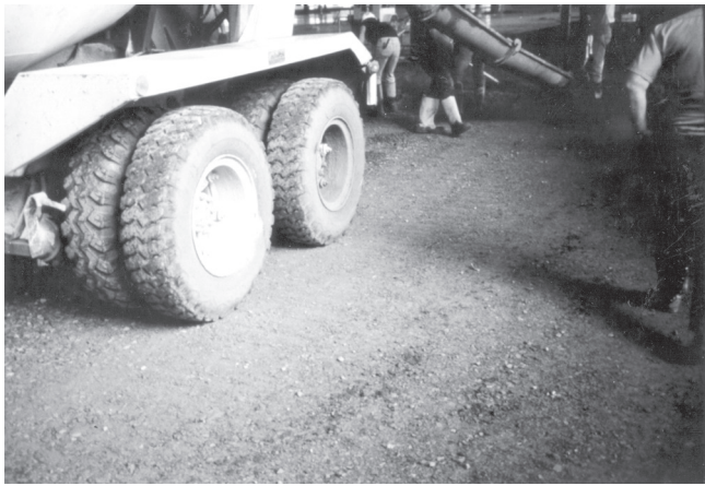
Fig. 6.1—Proof rolling by loaded concrete truck.
