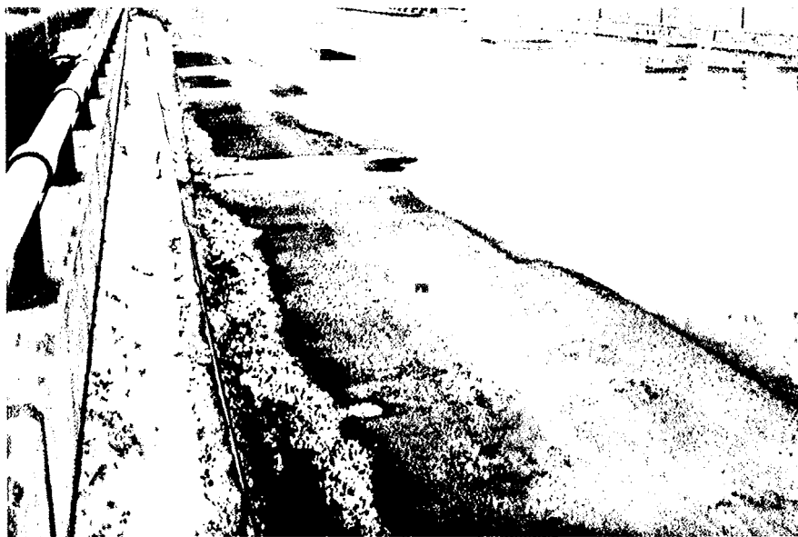
Fig. 17--Meltwater from the snow on the parapets keeps the bridge deck wet while the roadway (background) is dry
