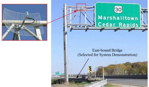
Figure 6 – Wireless communication equipment installed at the west end of the bridge.
