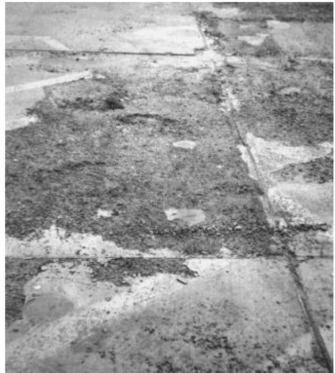
Fig. 3.1—Scaling is deterioration of concrete surfaces usually caused by exposure to freeze-thaw cycles.
