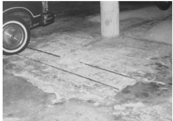
Fig. 3.2—Corrosion of reinforcement can lead to deterioration of concrete surfaces.
