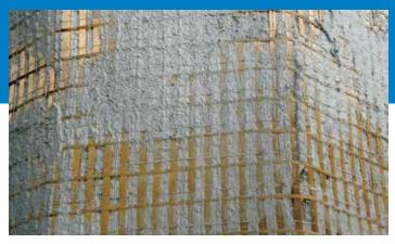
Composites with Inorganic Matrix for Repair of Concrete and Masonry Structures
