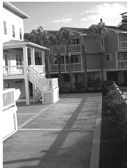
Fig. 3.1—Parking lot built with pervious concrete pavement.
