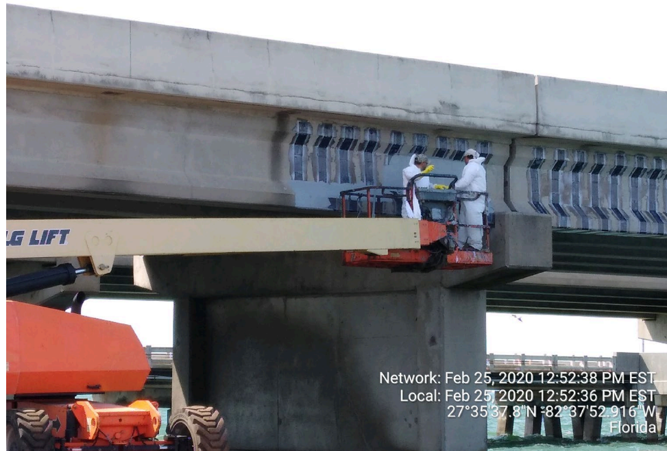
Fig. 17 —CFRP Wrap Installation
