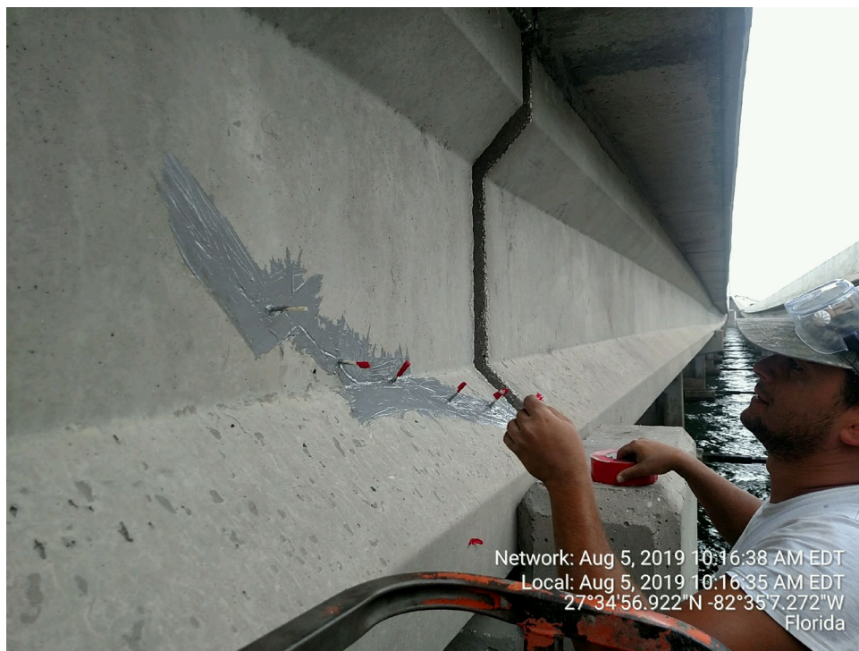
Fig. 16 —Surface Preparation: Epoxy Injection of Cracks
