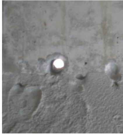
Fig. 21 —Hole for Mechanical Anchor
