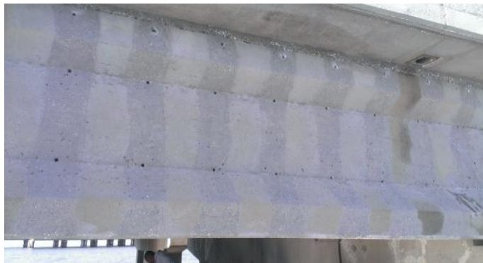
Fig. 22 —Surface Preparation with Holes for Mechanical Anchors
