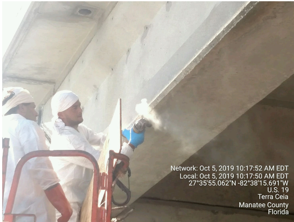
Fig. 15 —Surface Preparation: Smoothing Surface and Rounding Corners
