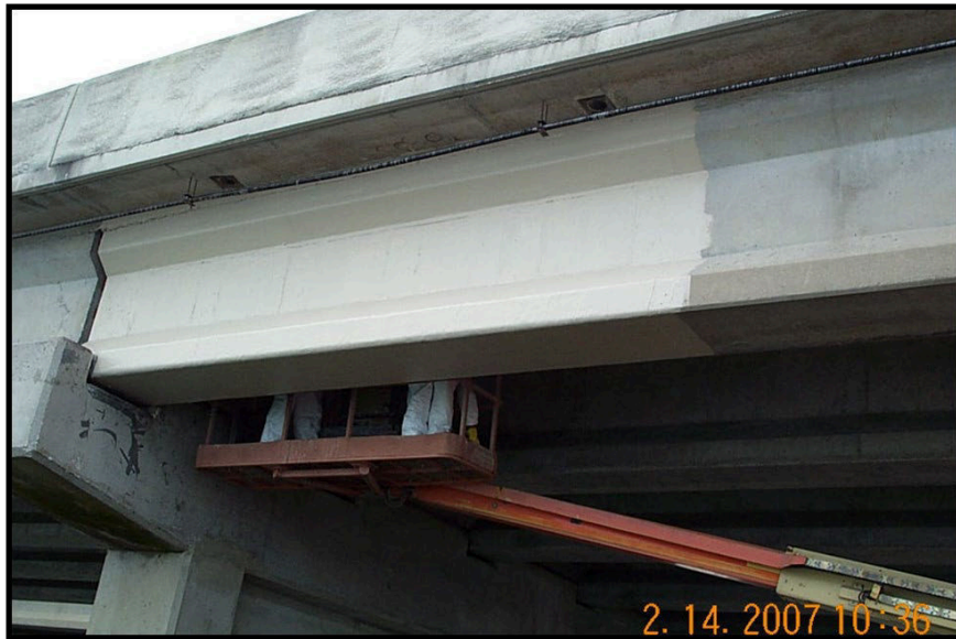
Fig. 20 —UV Coating over CFRP Wrap
