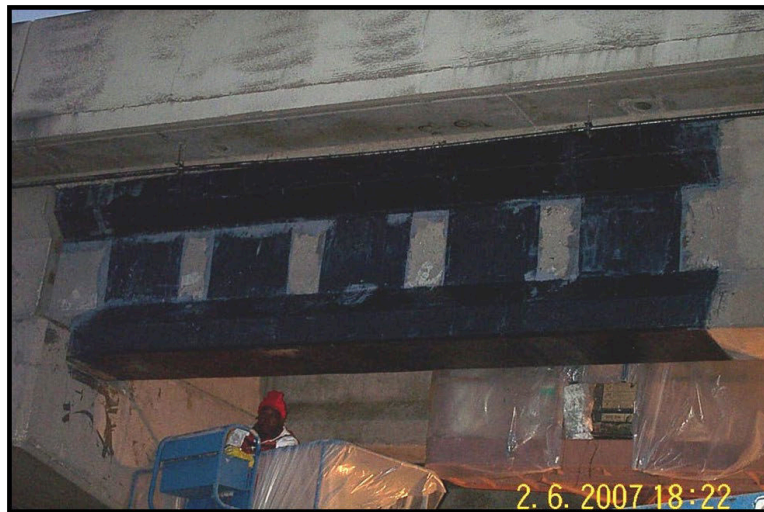
Fig. 18 —CFRP Wrap Installation in First Project Using Longitudinal CFRP Strips for Anchoring
