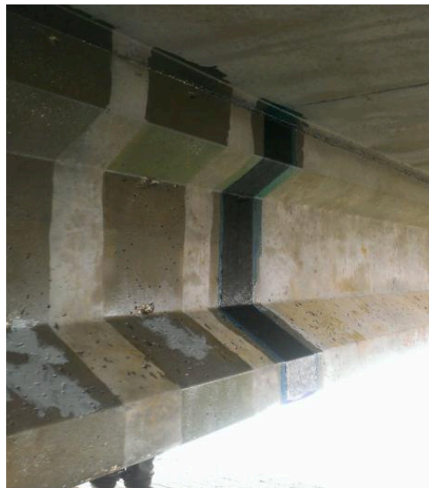
Fig. 23 —CFRP Installation over Mechanical Anchor Holes
