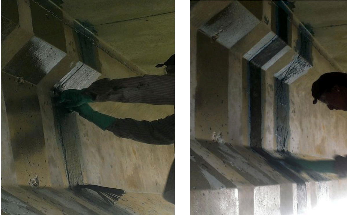
Fig. 24 —Fanning of CFRP Mechanical Anchors
