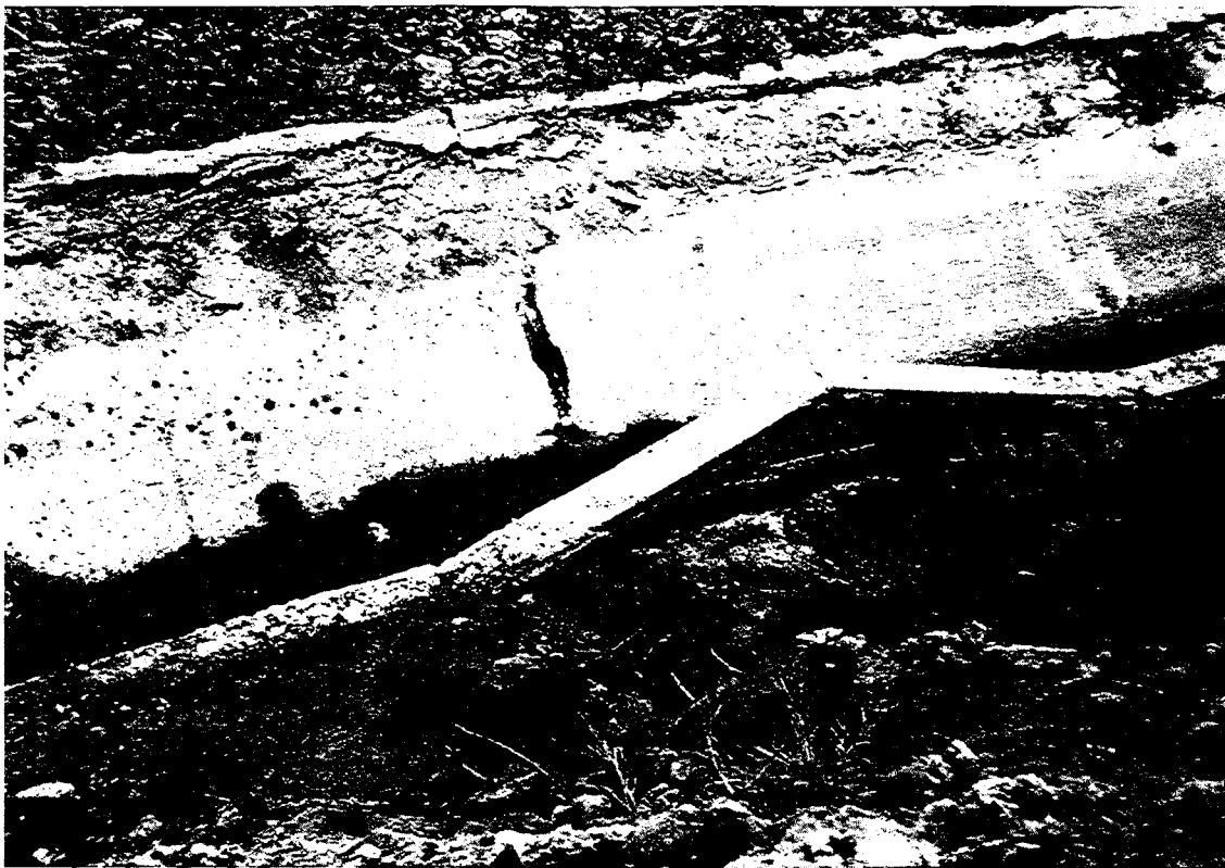
Fig. 2--Sulfate attack on concrete canal lining. San Luis Unit, Central Valley Project, California
