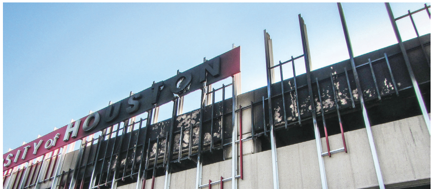
Fig. 3—Fire damage at exterior of garage
