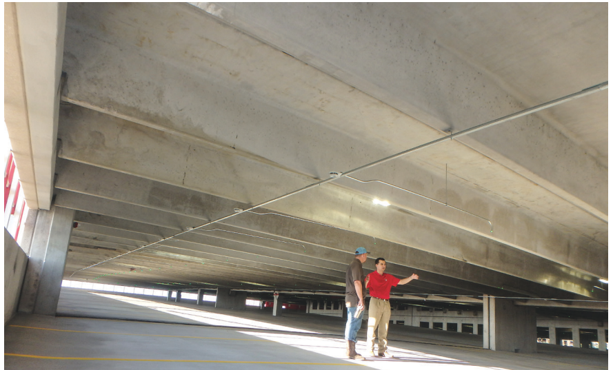
Fig. 8—New replacement double-tee beams at completion
