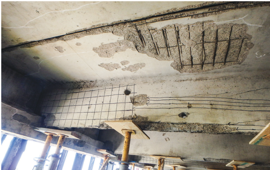
Fig. 6—Concrete cracking and spalling due to fire
