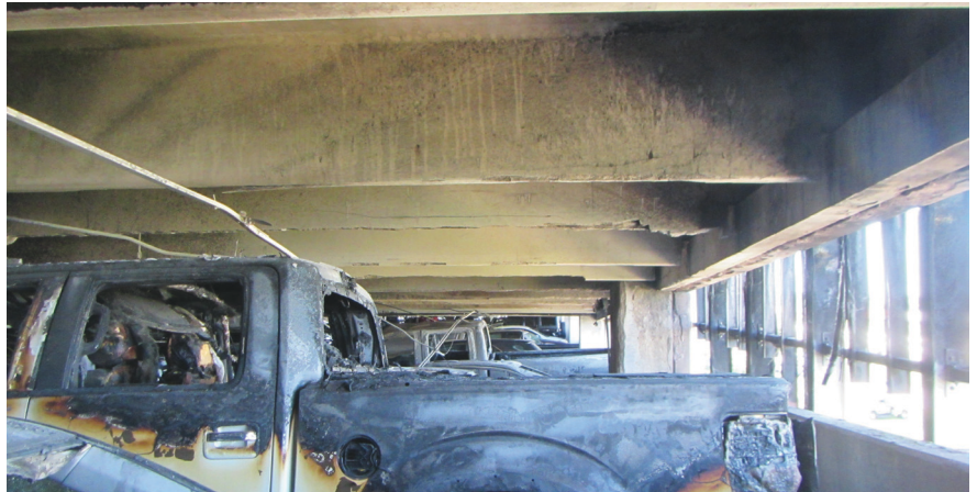
Fig. 2—Fire damage on Level 3 of parking garage
