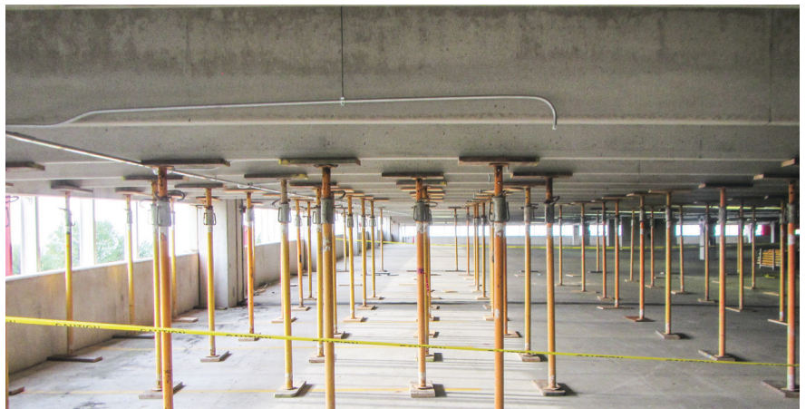
Fig. 4—Shoring installed in affected areas
