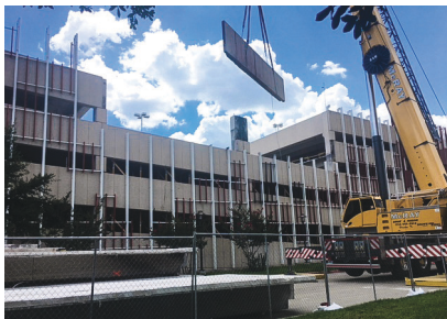
Fig. 7—Spandrel beam replacement
