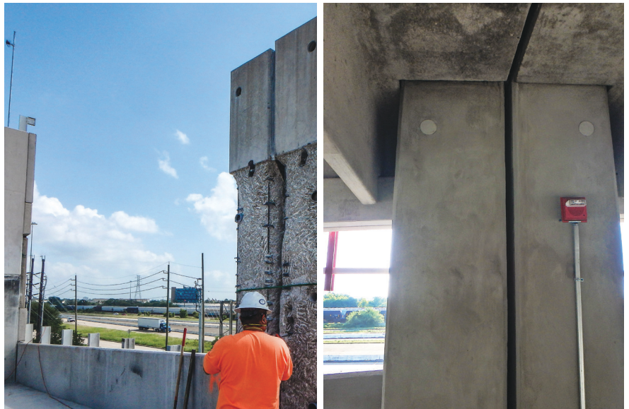
Fig. 9—Column during repair (left) and after repair (right)
