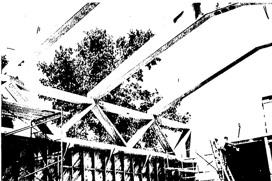
Fig. 9-2—Gravity Connection: A-frames bearing on precast trusses
