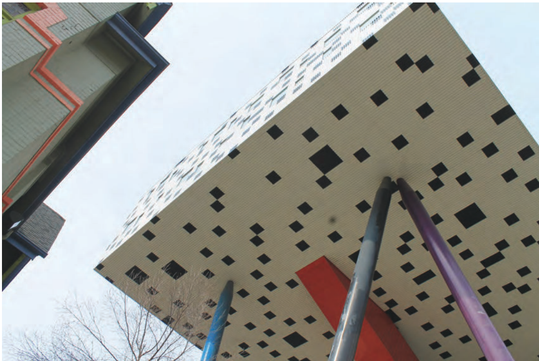
AESS columns with welded cast steel nodes at a university project in Toronto.
