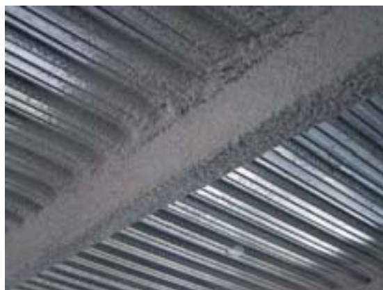
Fig I.1 Beam protected with SFRM.
