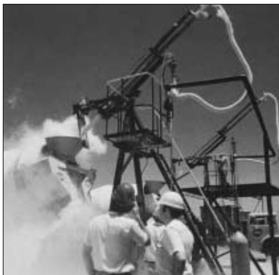
Figure 12.5 Injection of liquid nitrogen into an agitator truck to lower concrete temperature
