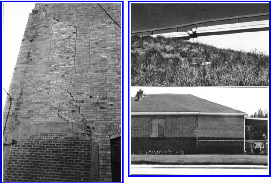
**Photograph 2. Photographs of damaged structures resulting from collapsible soils**
