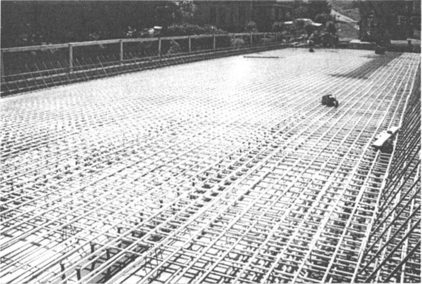
Figure 1. FRP Rebars in Concrete Bridge Deck - McKinleyville Bridge
