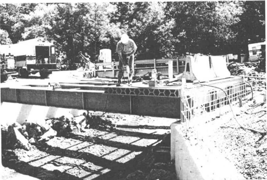
Figure 2. FRP Composite H-Deck (Superdeck™) - Wickwire Run Bridge
