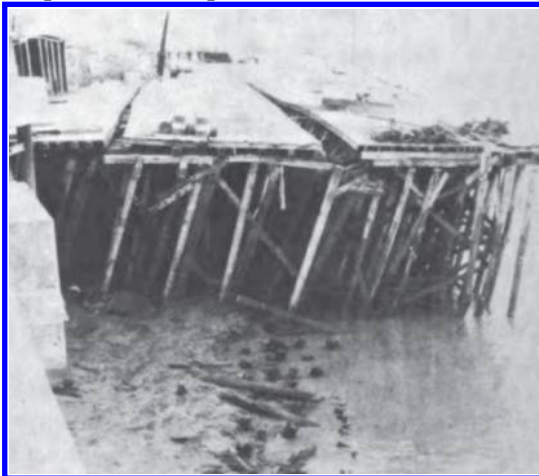
c) Leaning timber plumb pile structure partially demolished [Committee on the Alaska Earthquake 1973]
