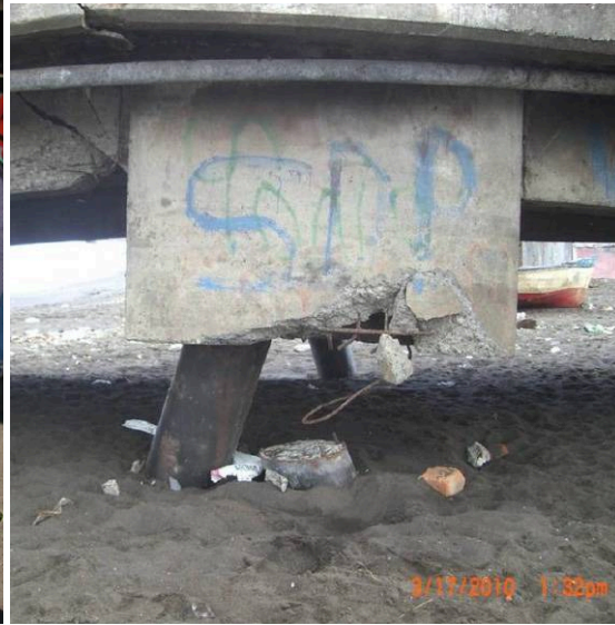
b) Ruptured connection at batter pile [GEER 2010]
