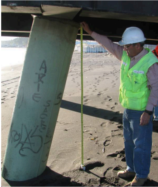
a) Formerly plumb steel pipe pile [ASCE 2013]
