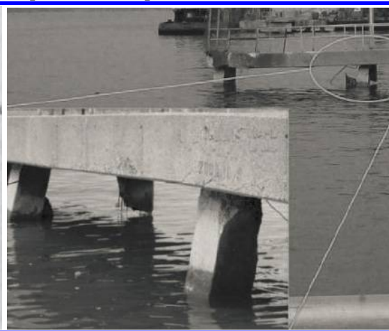
d) Formerly plumb concrete pile in Haiti [TCLEE 2012]
