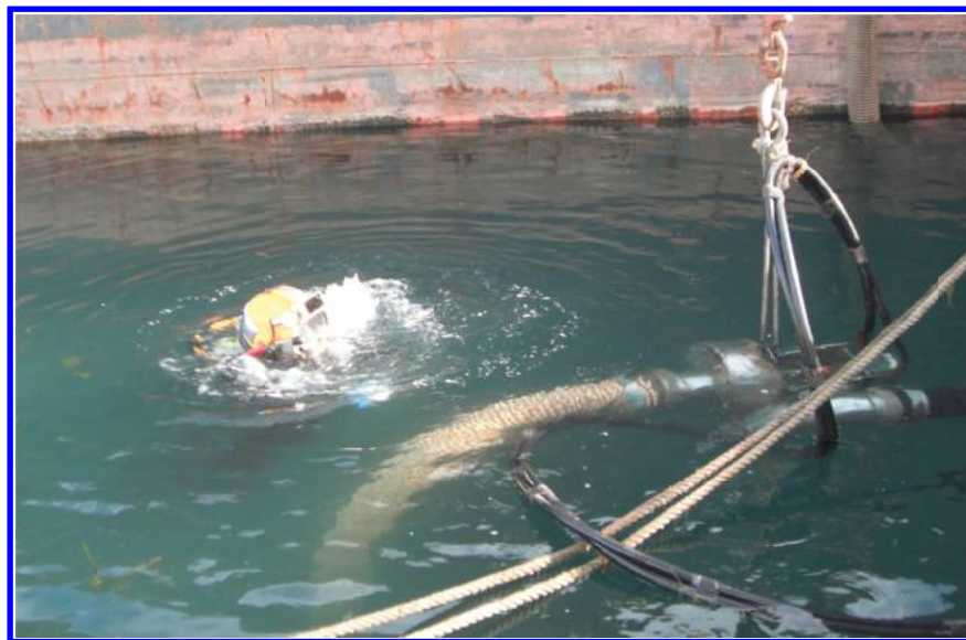
Figure 2-1. Diver-assisted Hydraulic Dredging System Using a System of a Cutterhead Dredge and Hoses.
