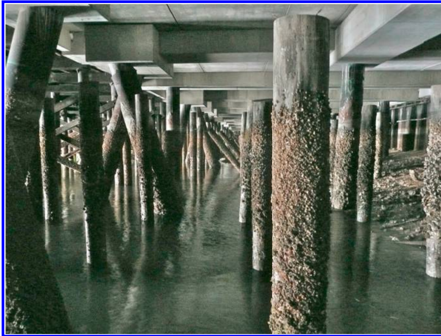
Figure 1. Typical Under-structure Conditions, Including a Series of Piles, Batter Piles, Timber Lagging, and Shoreline
