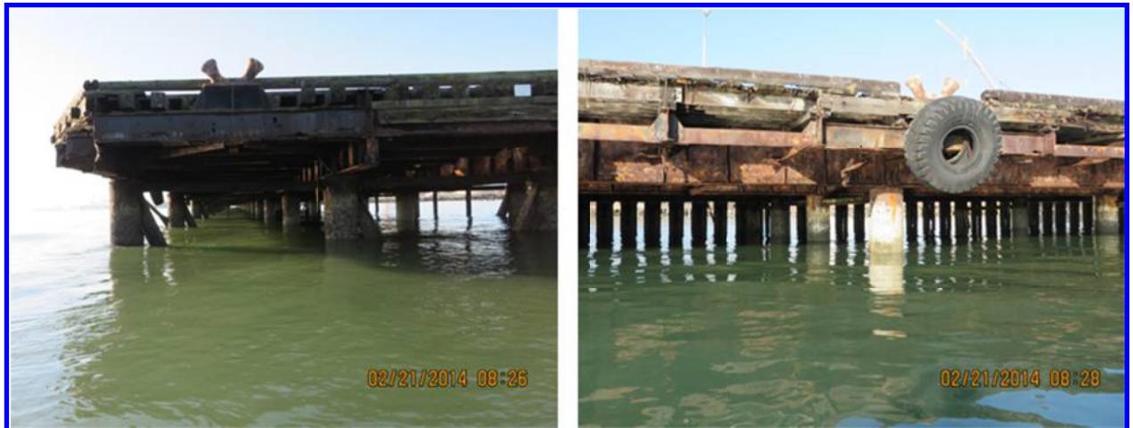
Figure 6. View from north end of Wharf 8 looking south (left) and timber screen on Wharf 8 (right), looking west.
