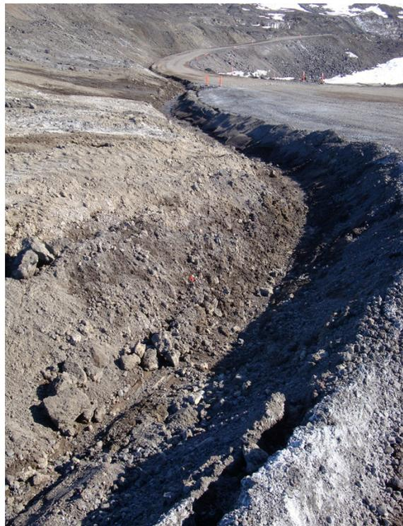
Figure 2. Upslope drainage ditches along the land transition of the SBT.
