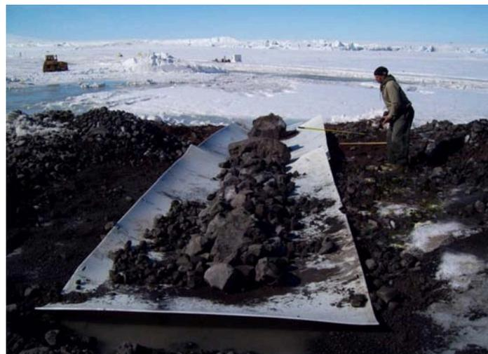
Figure 4. The fines and plastic are installed and large rock is placed along the center of the drain, 2010 construction.
