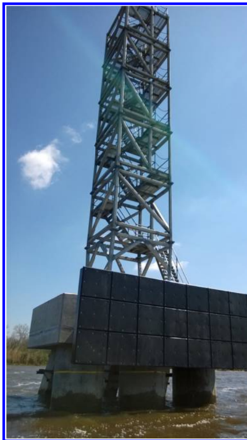
Photo 3. Catwalk and Stair Tower in Berth 1 (South Pier)
