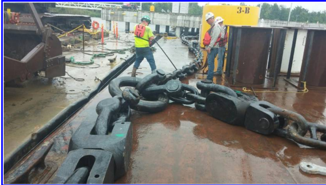
Photo 2. Fabricated Buoy and Anchor Chain Ready for Installation
