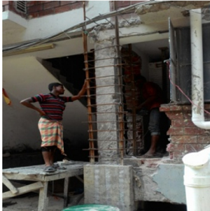
Reinforcement Arrangement for Column Jacketing
