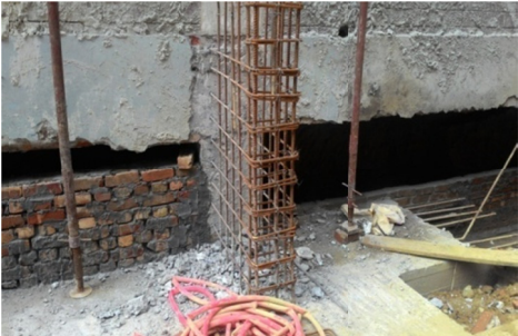
Reinforcement Arrangement for Shear wall
