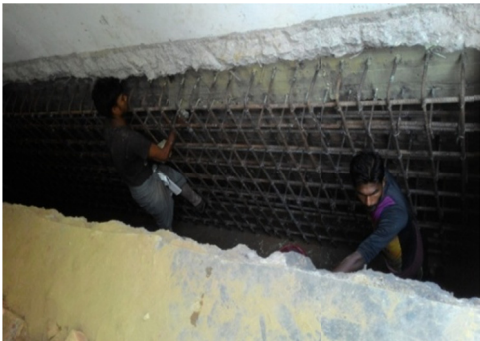
Reinforcement Arrangement for Deep Beam
