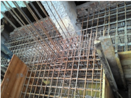
Reinforcement Arrangement for Deep Beam and Pile Cap
