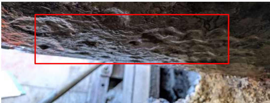
Figure 10. Wall loss defect validated by the City of Vancouver
