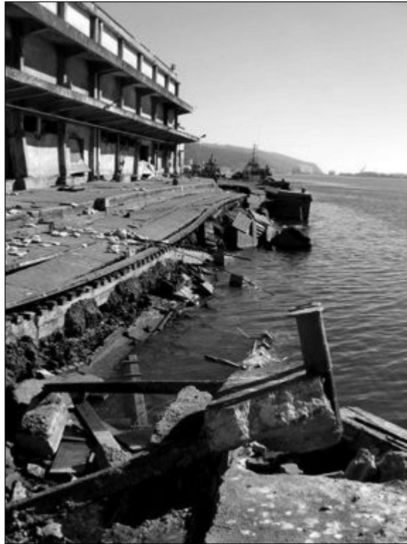
Figure 1.1 Damage to the Waterfront Observed in Talcahuano
