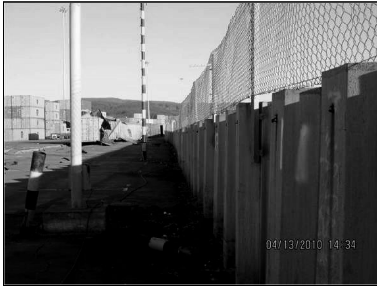
Figure 4.61 Steel Sheet Piles Adjacent to Beach with Lateral Spreading in Backlands
