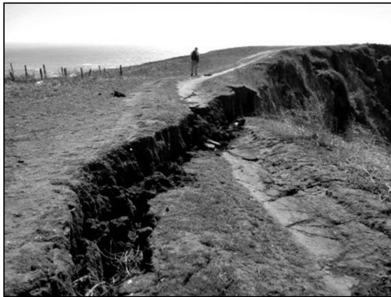
Figure 4.64 Earth Slope Failure on the Island North Point, Looking North
