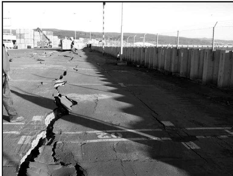
Figure 4.62 Lateral Spreading in the Backlands, Adjacent to the Beach Sheet Pile Structure
