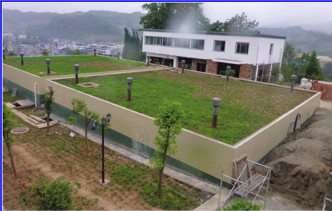
Figure 5-3. Two partially buried clearwells
