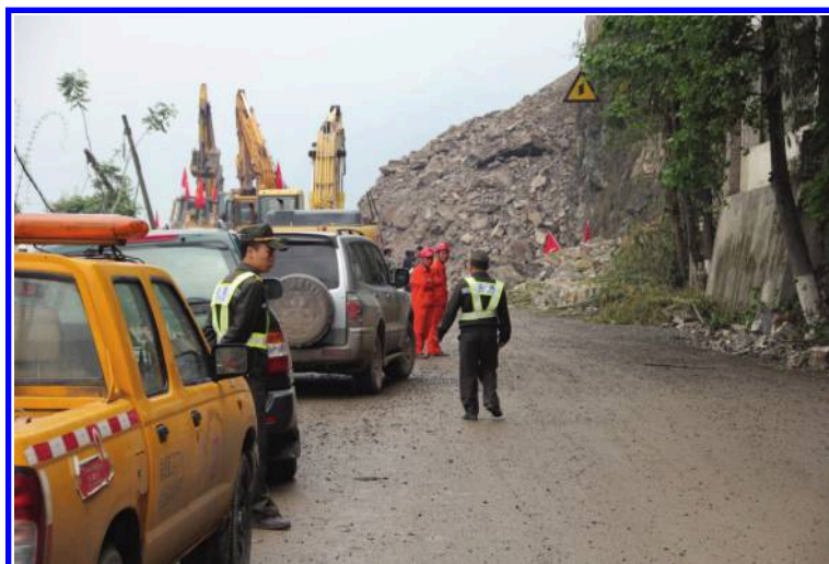
Figure 7-4. S210 Ling Guan Road damaged and blocked from landslide debris (Courtesy Dr. LIU Aiwen of CEA)
