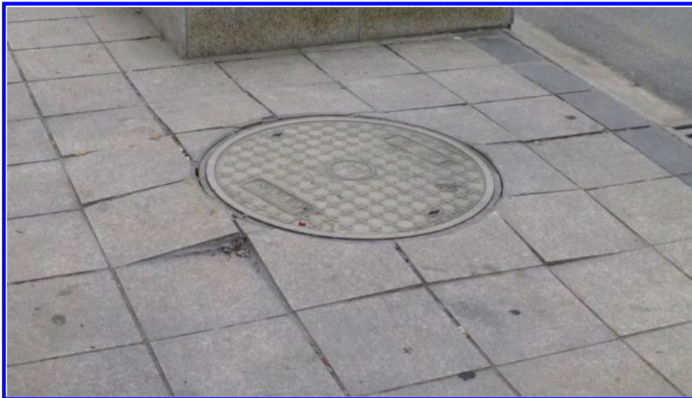
Figure 6-1. Floated manhole
