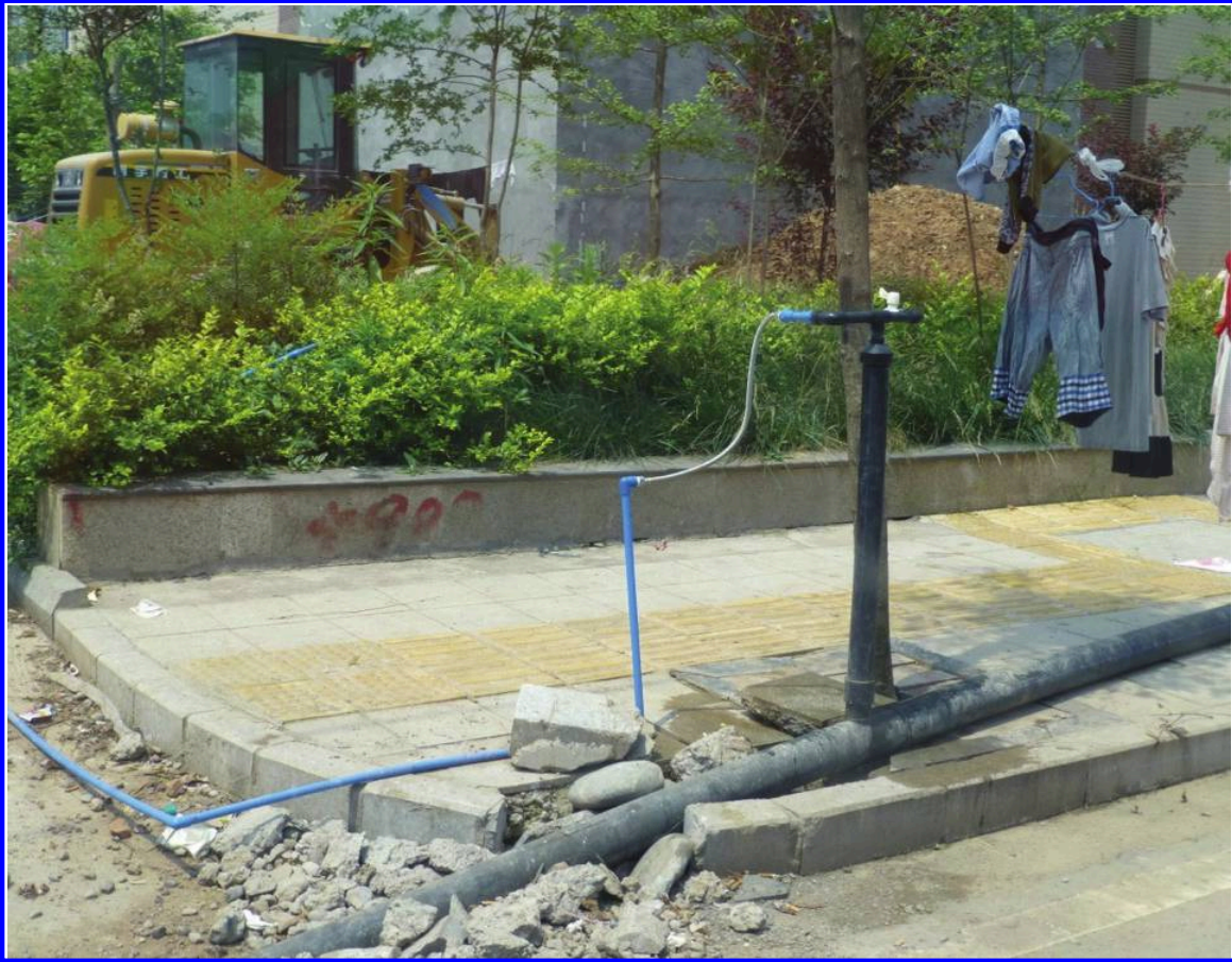
Figure 5-8. Above ground temporary water pipe
