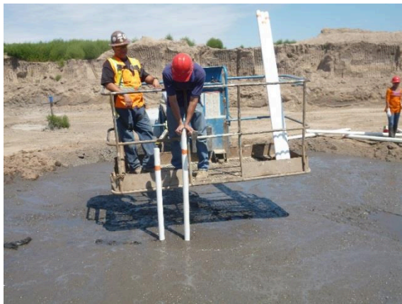
Figure 2. Installation of sampling pipes in the stabilized soil.
