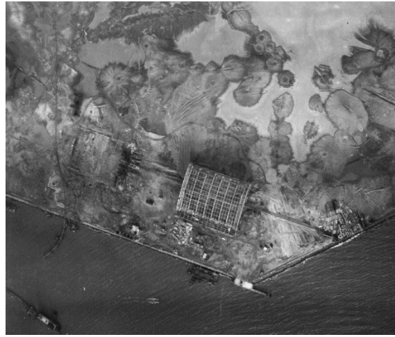
Figure 2. Construction Photograph: Early stages of hydraulic filling (February 1936) showing distribution lines and sand cones emanating from nozzles in the lines as well as shallow pools between sand cones
