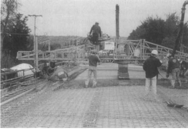
Fig. 6.3. Cast-in-place exodermic modules replaced decks of twin 600 ft bridges over Rt. 9W at Bear Mountain, NY.
