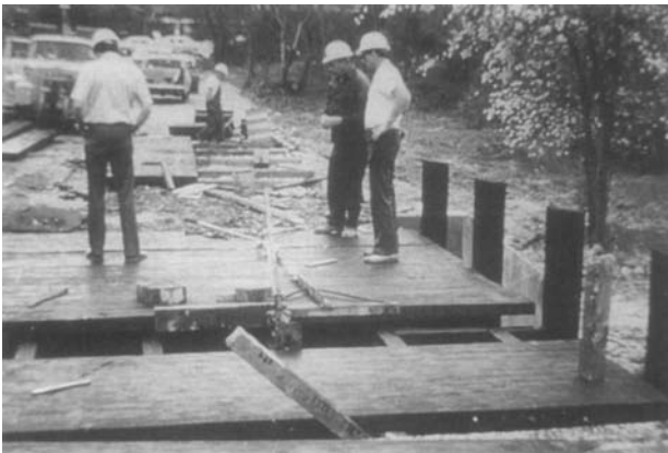
Fig. 6.5. Doweled glulam panels were field assembled to construct deck of all-timber bridge.
