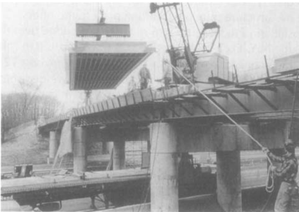
Fig. 6.2. Precast exodermic modules form the deck of bridge over New York State Thruway near Albany.
