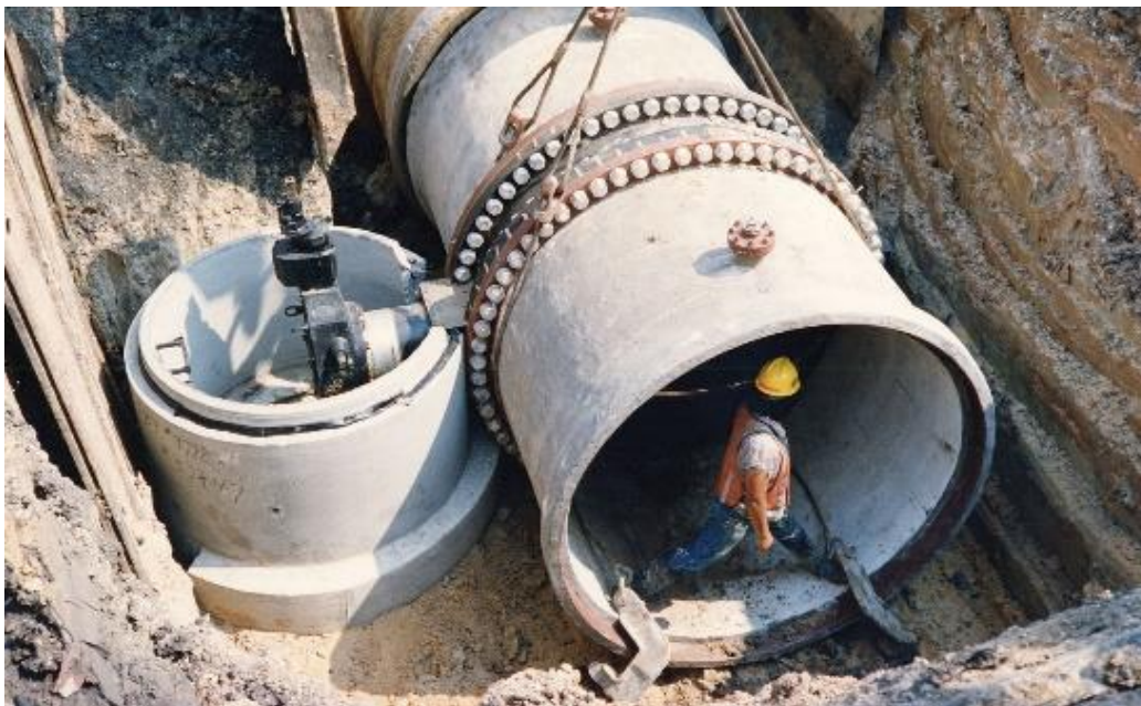
Figure 1: Typical Butterfly Valve Installation
